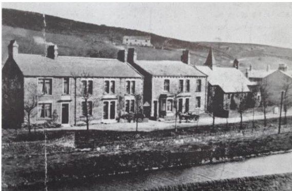
Photo 1. Quarry Road pre-1906 with the original Goit running between Brinscall and Withnell. The brick wall separating the Goit from Railway Rd can be seen at the bottom of the photo.
