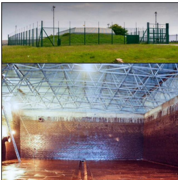
Photo 1. Pike Lowe upper reservoir, Brinscall.
