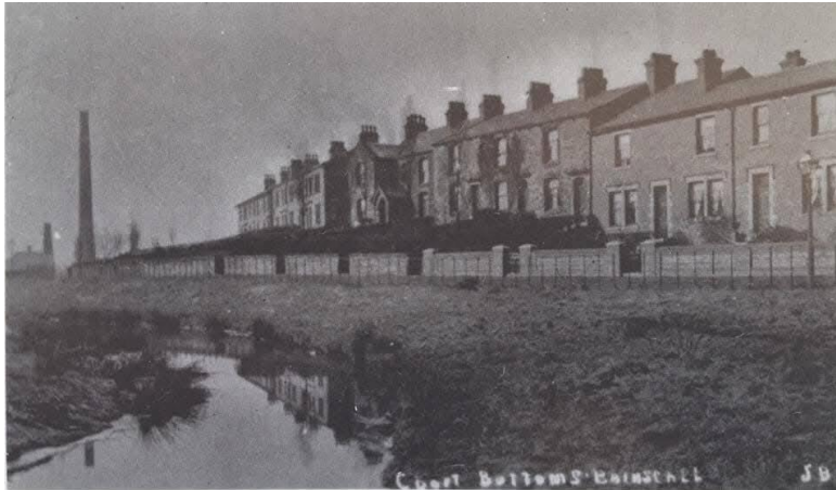
Photo 1. Croft Bottoms (Lodge Bank) – the factory complex can be seen in the background.
